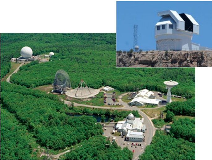
The tactical space situational awareness initiative is utilizing the Space Surveillance Telescope (above, inset) and the Haystack Ultrawideband Satellite Imaging Radar and Millstone Hill Radar (above) to demonstrate data fusion and sensor handoff approaches for improving the timeliness of the U.S. Space Surveillance Network, with the objective of achieving tactical command-and-control responsiveness.
